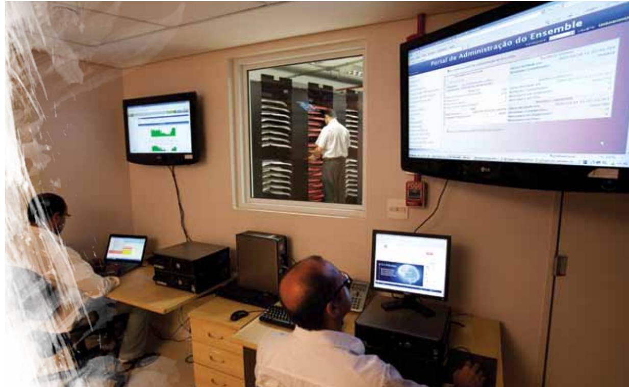
Installation of the new datacenter
